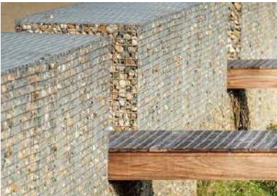
HA-HA WITH BRIDGE ACCESS
