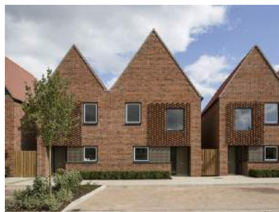
VARIED ROOFSCAPE ON SEMI-DETACHED HOUSES
