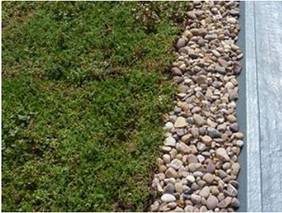
BROWN / GREEN ROOF
