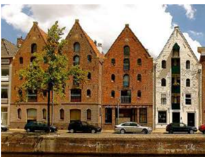
A VARIETY OF ROOF FORMS AND MATERIAL TREATMENTS FOR LARGER BUILDINGS
