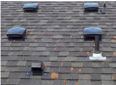
VISIBLE ROOF PENETRATIONS
