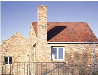
PRINCIPAL MATERIAL TAKEN THROUGH ENTIRE BUILDING
