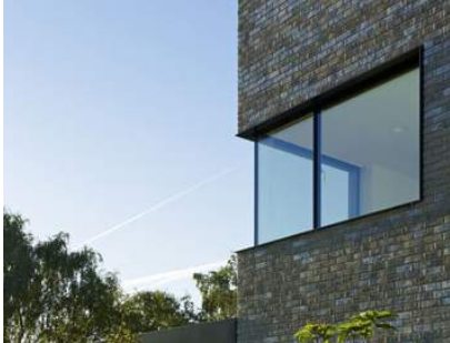
RECESSED CORNER WINDOW WITH SLENDER FRAME SECTION
