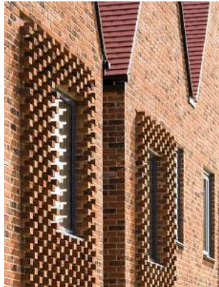
DETAILING ADDS TEXTURE AND HELPS TO DEFINE OPENINGS IN A FACADE
