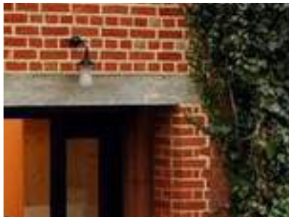
CONCRETE LINTELS ABOVE DOORWAYS
