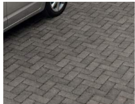
CONCRETE BLOCK HERRINGBONE RAISED TABLES AND SHARED SURFACES
