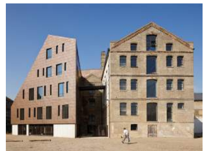
LARGER FOOTPRINT BUILDINGS WITH VARIED ROOF FORMS
