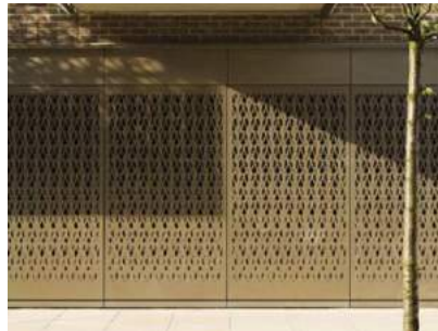
EXAMPLE OF AN INTEGRATED BIN STORE IN AN APARTMENT BUILDING WITH VENTILATION SCREENS
