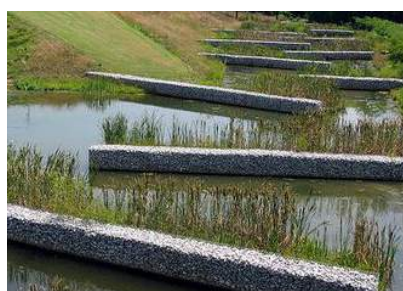
DETENTION BASIN BAFFLES
